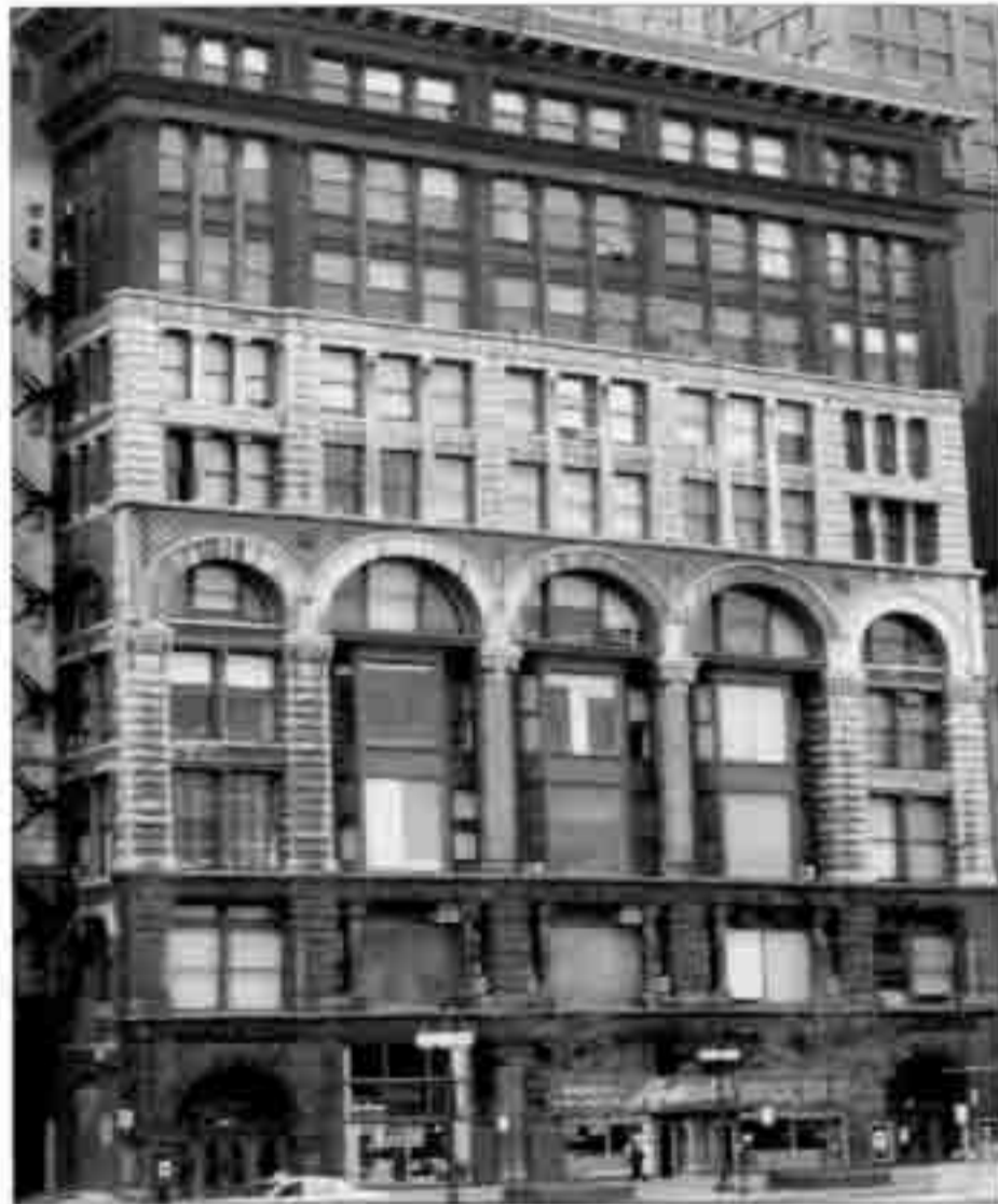
The Studebaker/Fine Arts Building. The arched doorways at street level on the left and right were originally entries for customers and their carriages to an interior drive. The top three stories were added during the 1896 renovation. The ground floor currently includes the Artist's Snack Shop, a fine eatery, and Bookseller's Row used book store.
