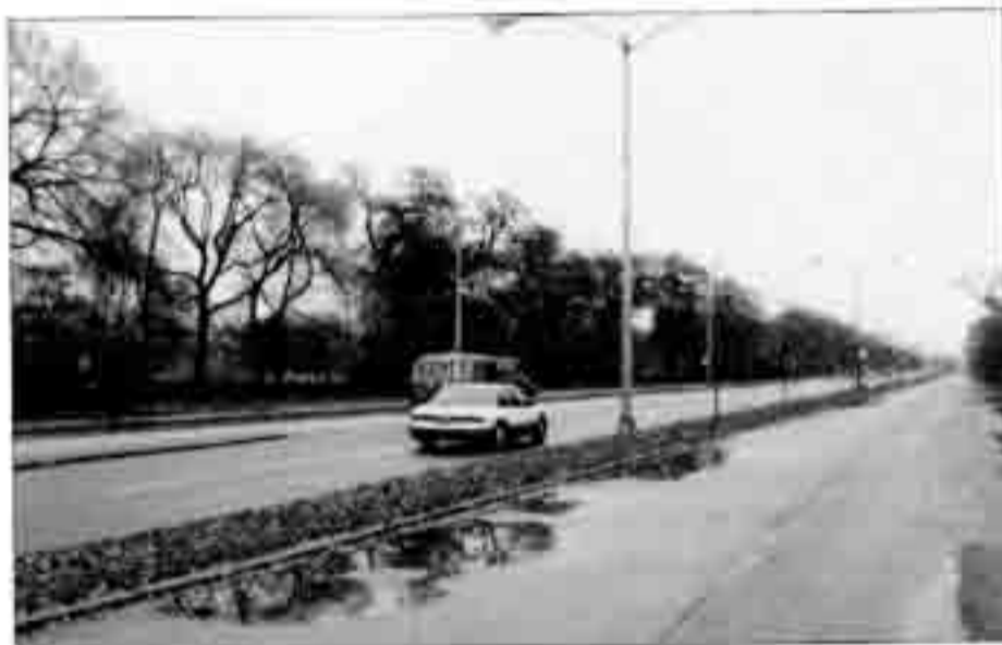
Two vehicles eastbound on the boulevard section of Ogden Avenue through Douglas Park. In the foreground are the "local" eastbound lanes. The main thoroughfare has 4 total lanes, two each direction. The local westbound lanes are on the far side of the road.
